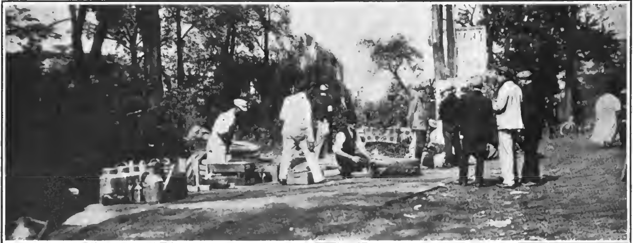
DIAMOND TIRE REPAIR STATION FOR AMERICAN CARS ON THE LAKEVILLE-HYDE PARK ROAD NEAR LAKE SUCCESS.
